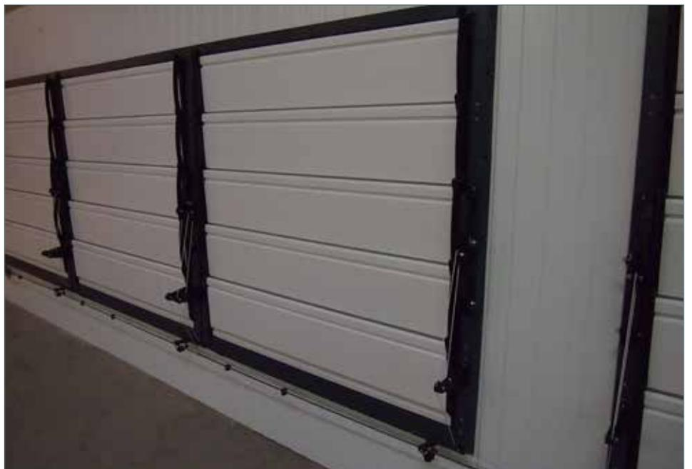
*Due to the insulated inlet flaps of the DA 17K tunnel inlet, cold areas are avoided in front of the inlet and the animals are given optimum conditions.*
